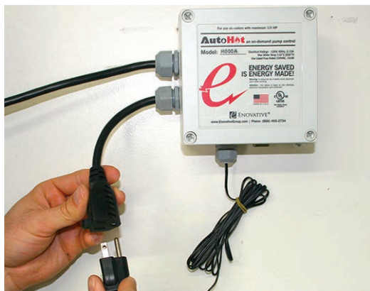
1. Unplug the recirculation pump from the AutoHot®
